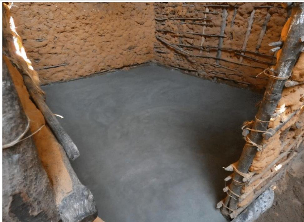
Halving the incidence of Tungiasis with tough, low cost flooring
